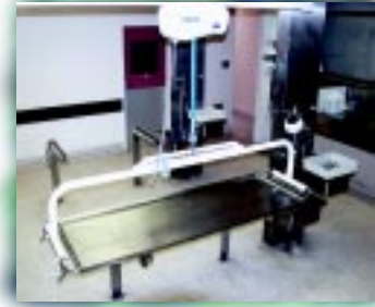
The Wispa Ceiling Mounted Hoist allows easy transfer to the Post Mortem Room
